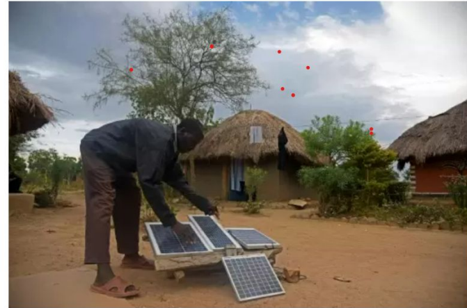
A resident setting his mini solar system for charging lights, phones and radios.
